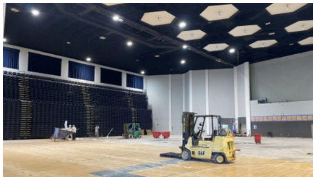
The Omni Auditorium under construction.
